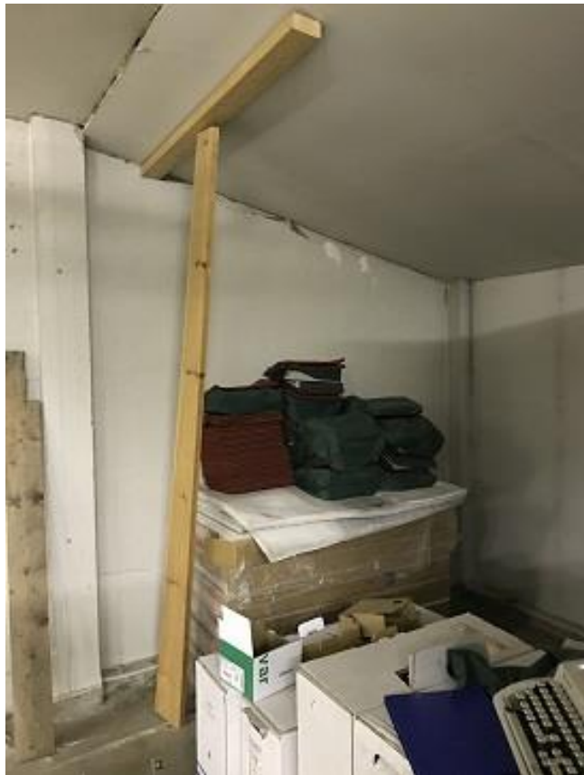
Fig. 6.2 – Skadet himling
