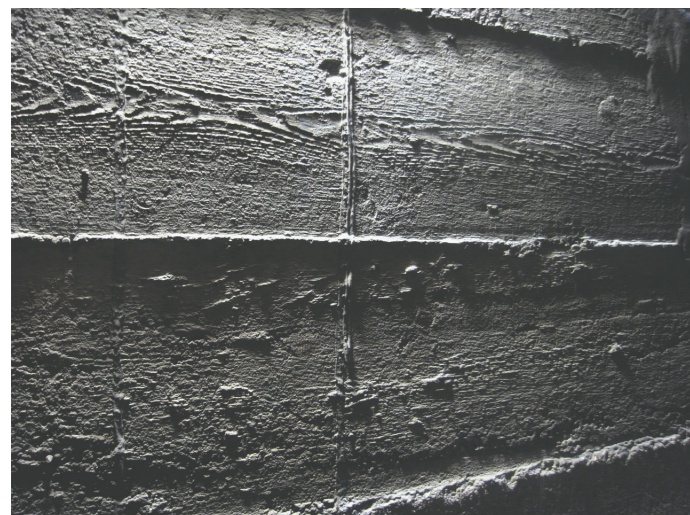
Beton-brut - grov overflate
