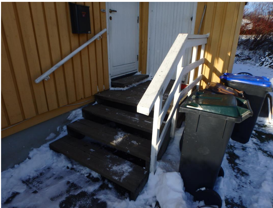
Figur 12: CCA-impregnert trapp.
