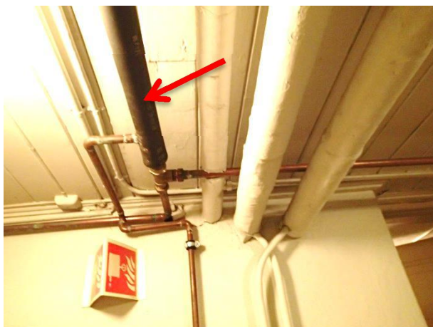
Bilde 14: Cellegummi in U.et.
