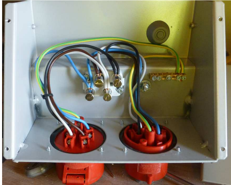
Figure 8: Detail of termination JB.
