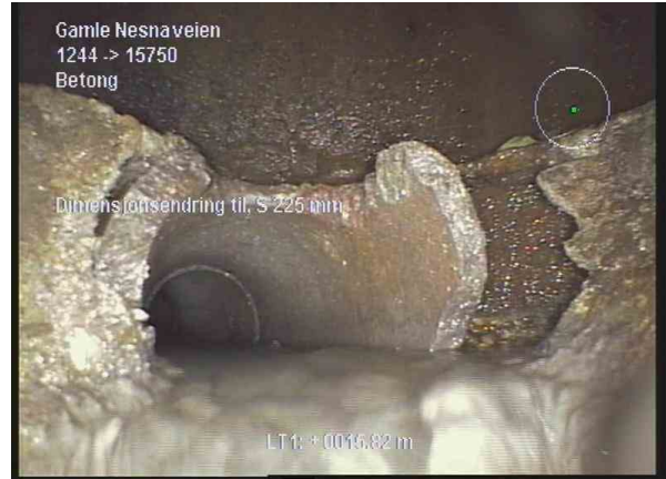
13.11.2024 144510_15750_1244_13112024_024601_038.jpg, 00:01:31, 15.80m Dimensjonsendring til, S 225 mm
