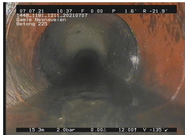
10, 00:03:58, 15.34m Materialendring til, Betong
