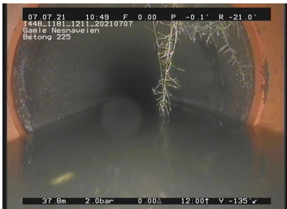
21, 00:08:41, 37.86m Materialendring til, Betong
