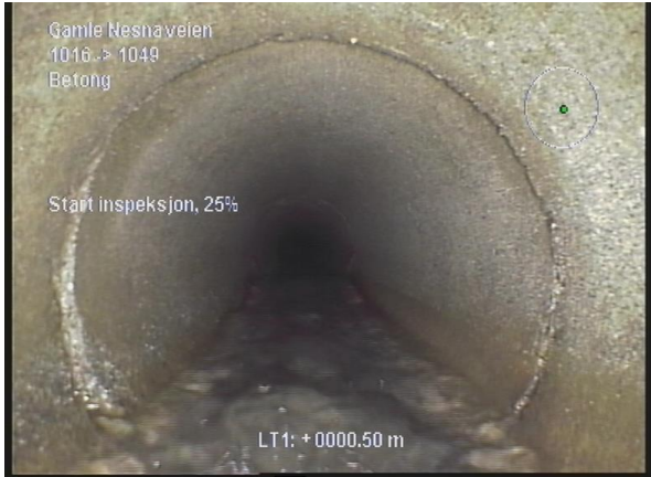
14.11.2024 150201_1016_1049_14112024_030307_040.jpg, 00:00:00, 0.50m Start inspeksjon, 25% / Rennende vann
