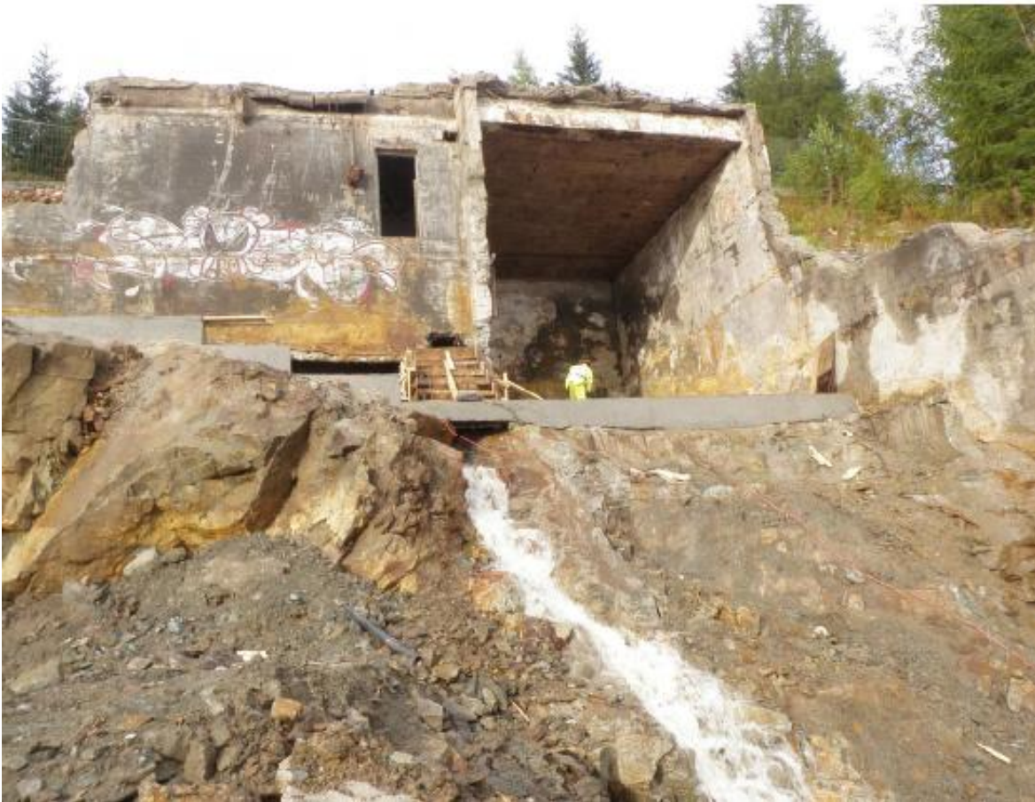
Figur 15 Killingdalbekken ledet under ny betongplate for Killingdalparken (Multiconsult, 2010).
