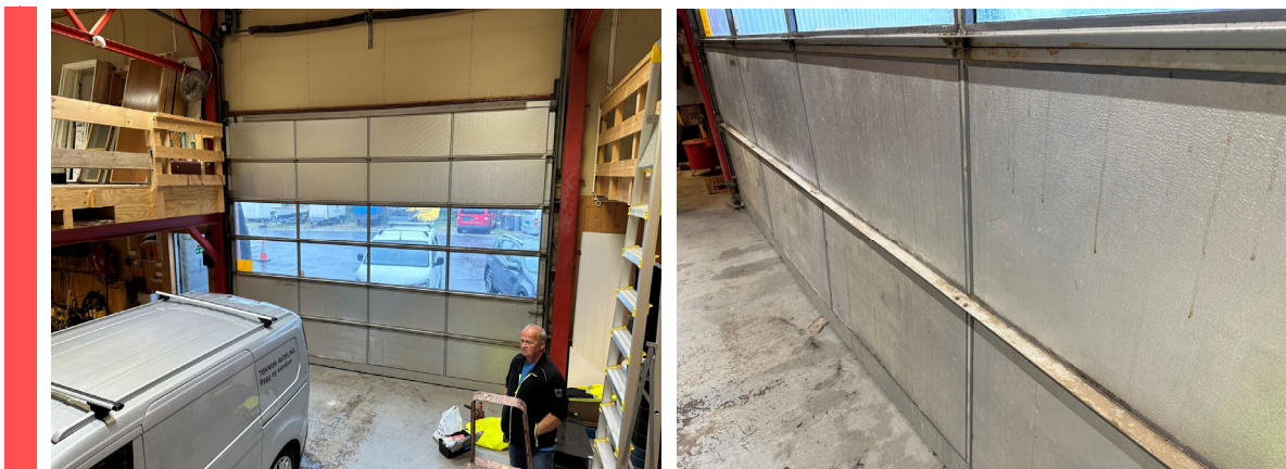
Figur 18 – Isolert leddport.
