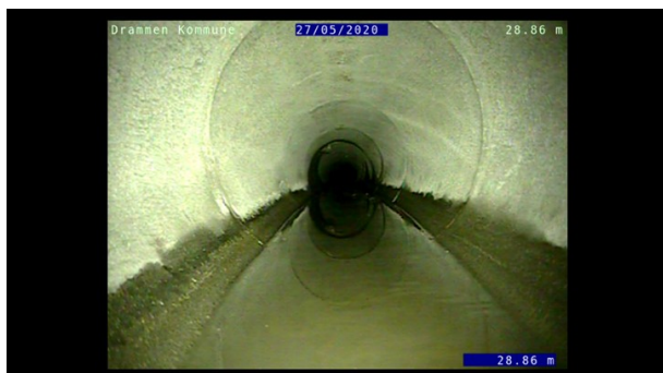
Foto: L22501_22161_22159_27052020_4_6_28,863_D.JPG, 00:02:35 28,86m, Vannivå 5%, Start
