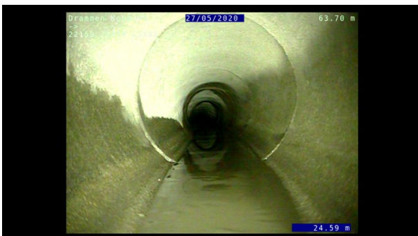
Foto: L22454_22159_22111_27052020_3_3_24,585_D.JPG, 00:02:36 24,58m, Vannivå 5%, Start
