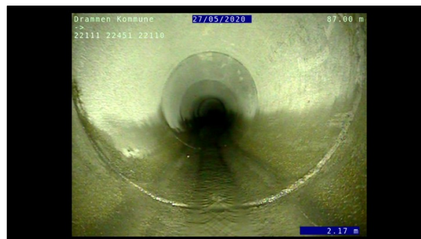
Foto: L22451_22111_22110_27052020_2_2_2,174_D.JPG, 00:00:24 2,17m, Vannivå 0%, 1
