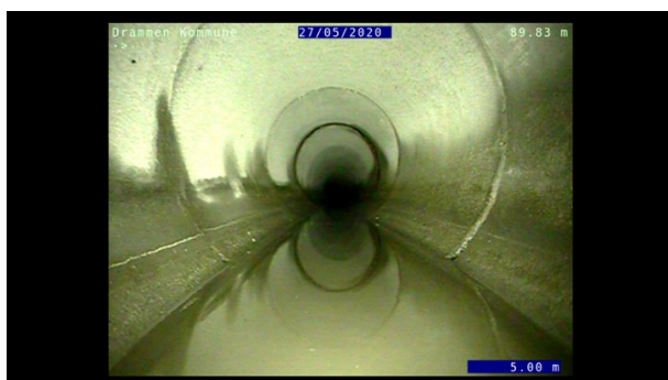
Foto: L22451_22111_22110_27052020_2_3_4,996_D.JPG, 00:00:50 5m, Vannivå 5%, Start
