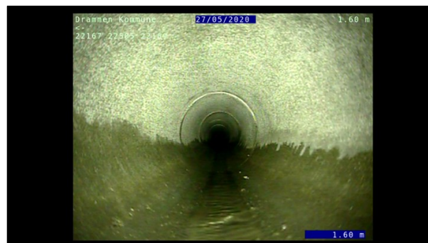
Foto: L22505_22169_22167_27052020_6_2_1,603_U.JPG, 00:00:22 1,6m, Vannivå 0%, 1%
