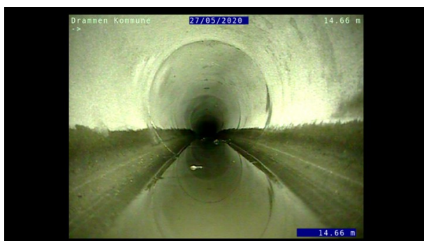
Foto: L22501_22161_22159_27052020_4_3_14,663_D.JPG, 00:01:07 14,66m, Vannivå 5%, Start
