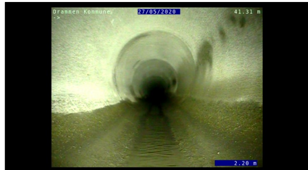
Foto: L22454_22159_22111_27052020_3_2_2,196_D.JPG, 00:00:28 2,2m, Vannivå 0%
