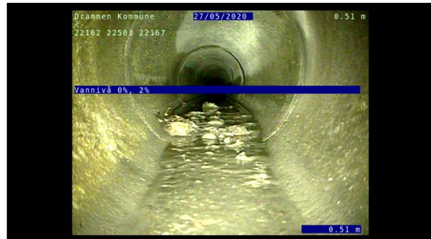
Foto: L22503_22167_22162_27052020_5_2_0,506_U.JPG, 00:00:04 0,51m, Vannivå 0%, 2%
