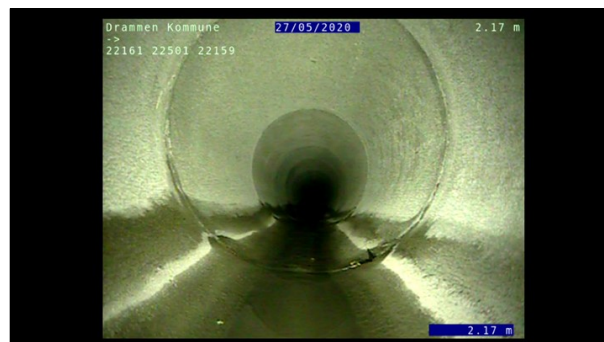
Foto: L22501_22161_22159_27052020_4_2_2,173_D.JPG, 00:00:21 2,17m, Vannivå 0%, 1%
