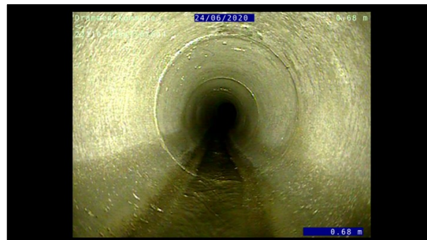
Foto: L67647_67644_22110_24062020_1_2_0,682_U.JPG, 00:00:57 0,68m, Vannivå 0%, 2%
