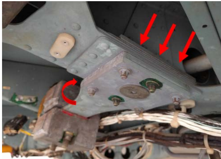
Figure 2. Location of A953-1 and A956 Assembly installation on aircraft hammer weight fitting
