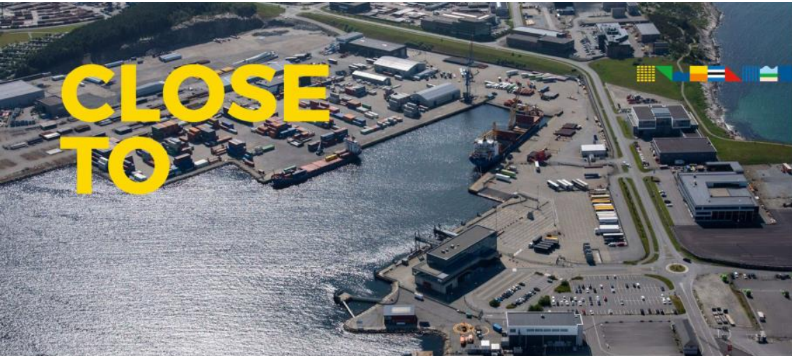
FTR – Ferry Terminal Risavika – Kameraovervåket
