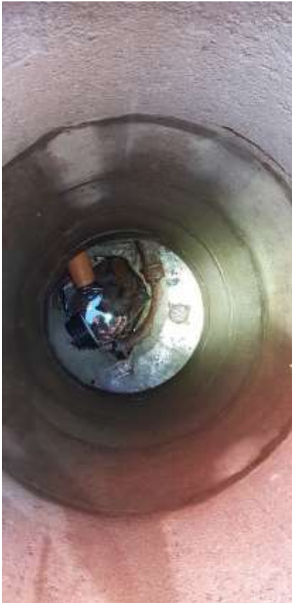
Ov kum 16100. Ende rørfornying
