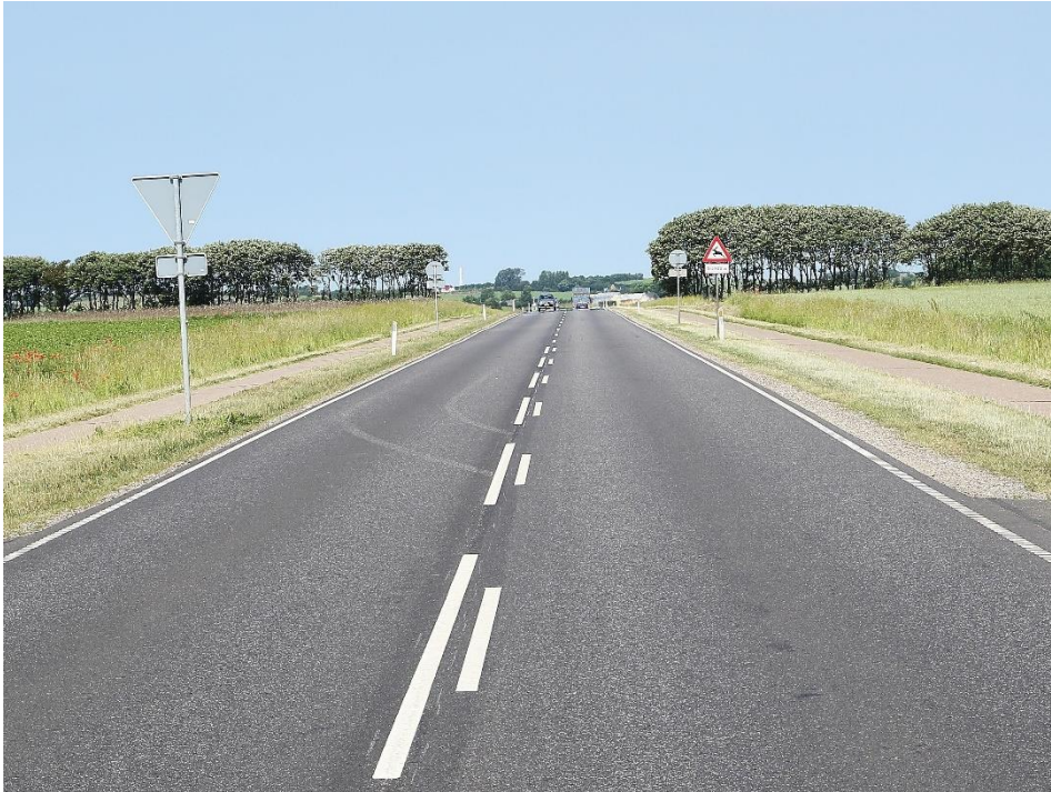
Figure 4. The road used for the Danish test site. (Photo: Trond Cato Johansen, Ramboll).
