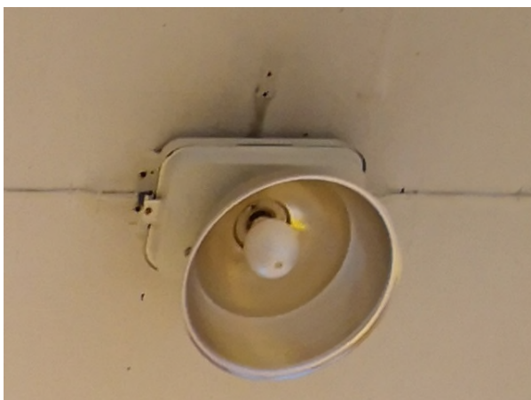
Figur 31: Gamle metallhalogen-armaturer
