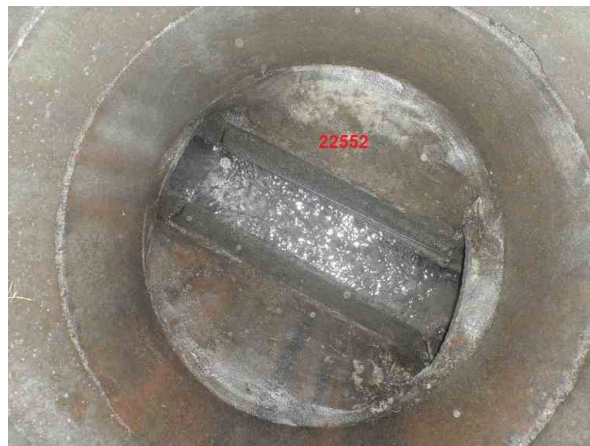
L_22551_22552__34.jpg, 00:00:00, 0.01m Start inspeksjon, 0%
