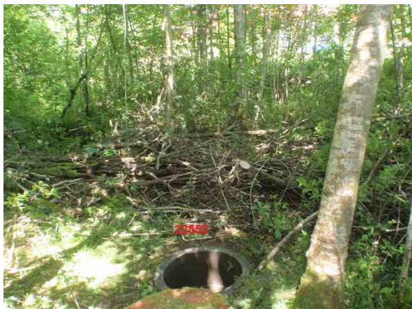
L_22551_22552__33.jpg, 00:00:00, 0.01m Start inspeksjon, 0%
