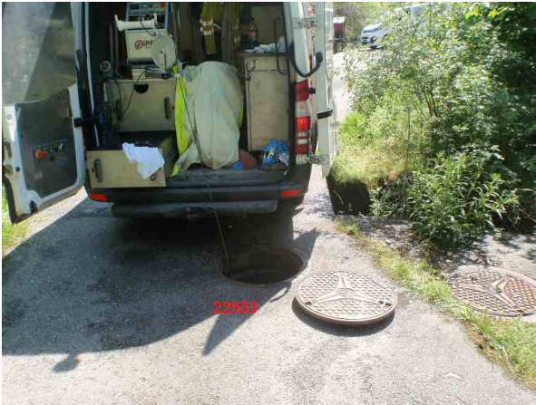
L_22552_22553__31.jpg, 00:00:00, 0.00m Start inspeksjon, 50%
