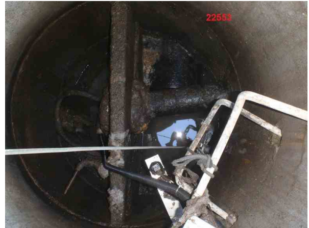
L_22552_22553__32.jpg, 00:00:00, 0.00m Start inspeksjon, 50%
