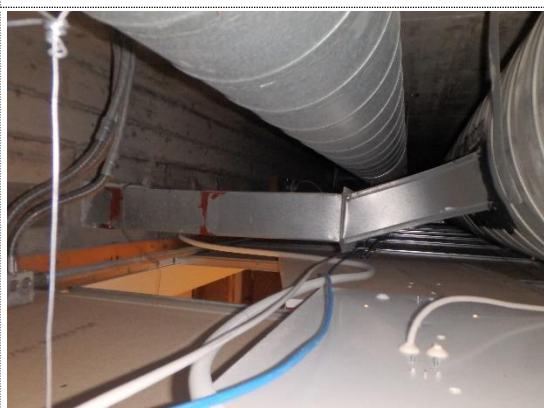
Over himling i korridor
