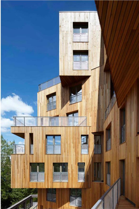
The Cube, London. Arkitekt: Hawkins\Brown, foto: Jack Hobhouse kilde: www.archdaily.com
