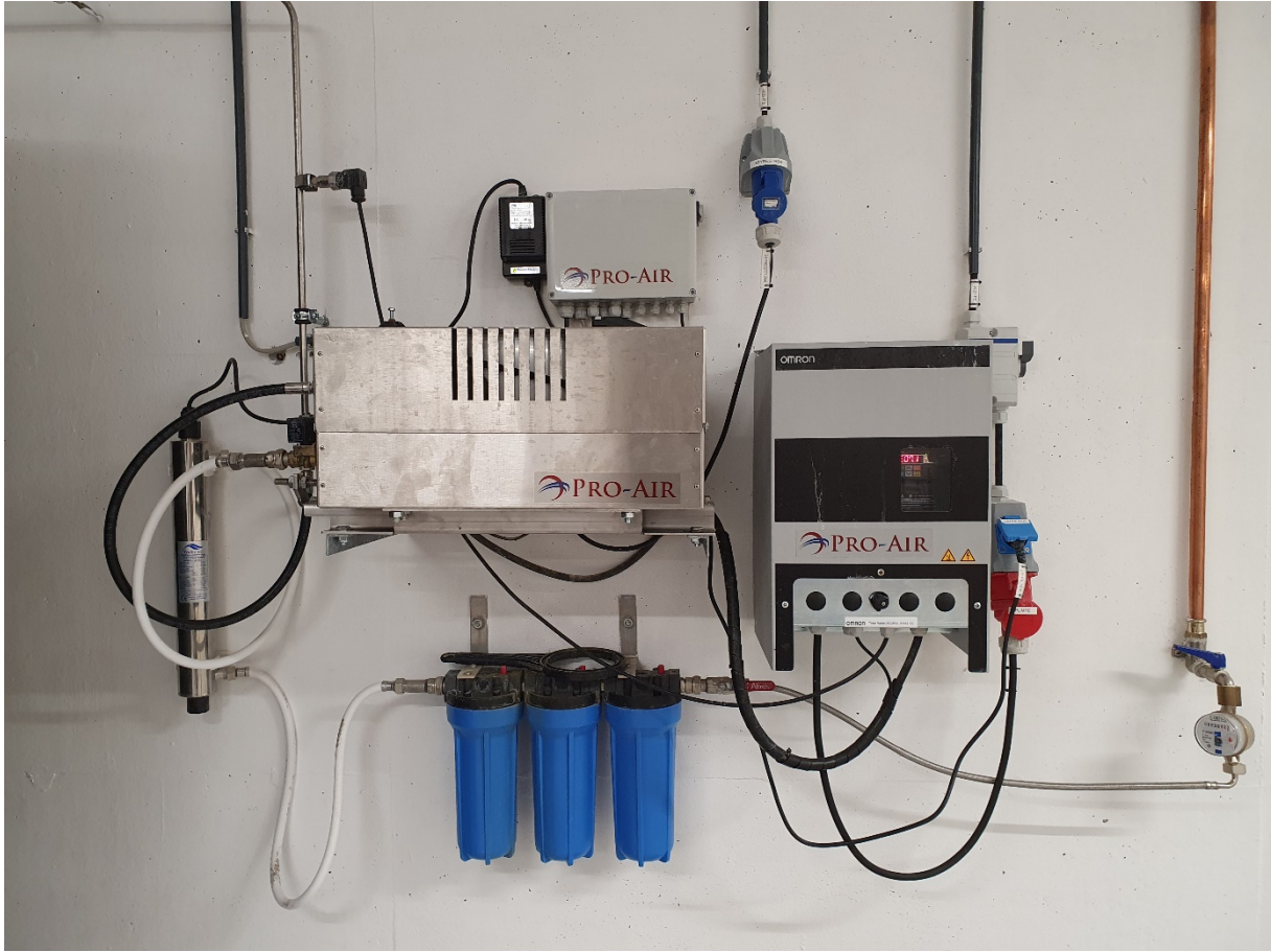
Picture 1. Existing high-pressure humidification unit in the technical rom
