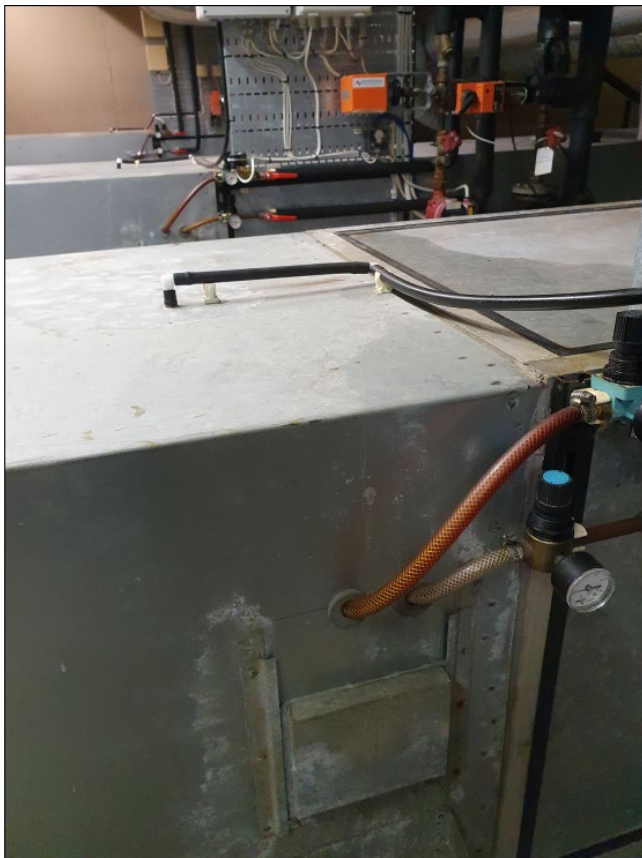
Picture 5: the black tube puts CO2 in the cabinet and the white and red tube is used for the existing humidity system (white is air and red is water). These 2 last ones must be replaced by the new high-pressure humidity system
