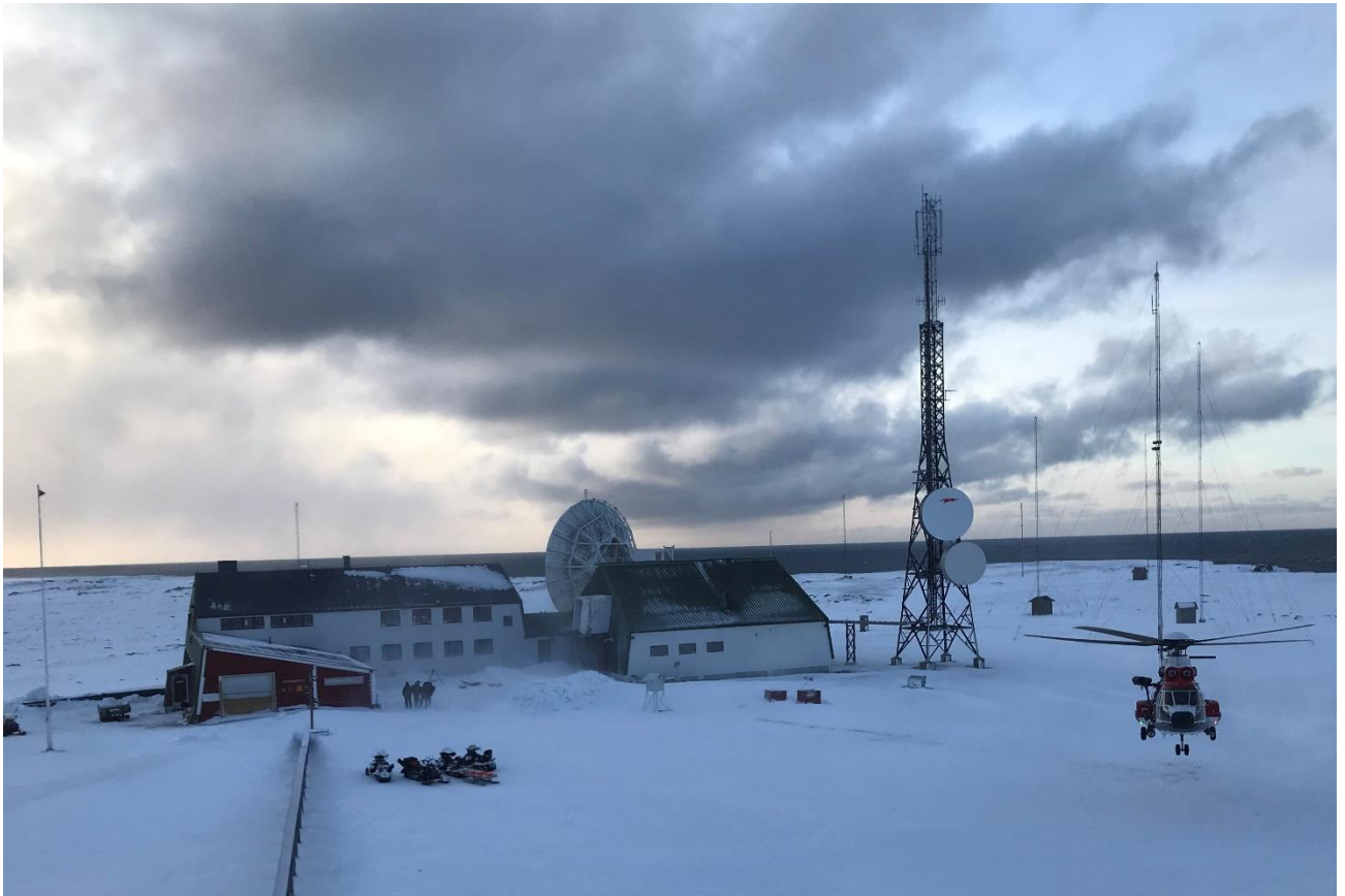
Figure 2 Isfjord Radio main building. The location of the battery will be in the building between the big parabola and the antenna. Photo: Multiconsult
