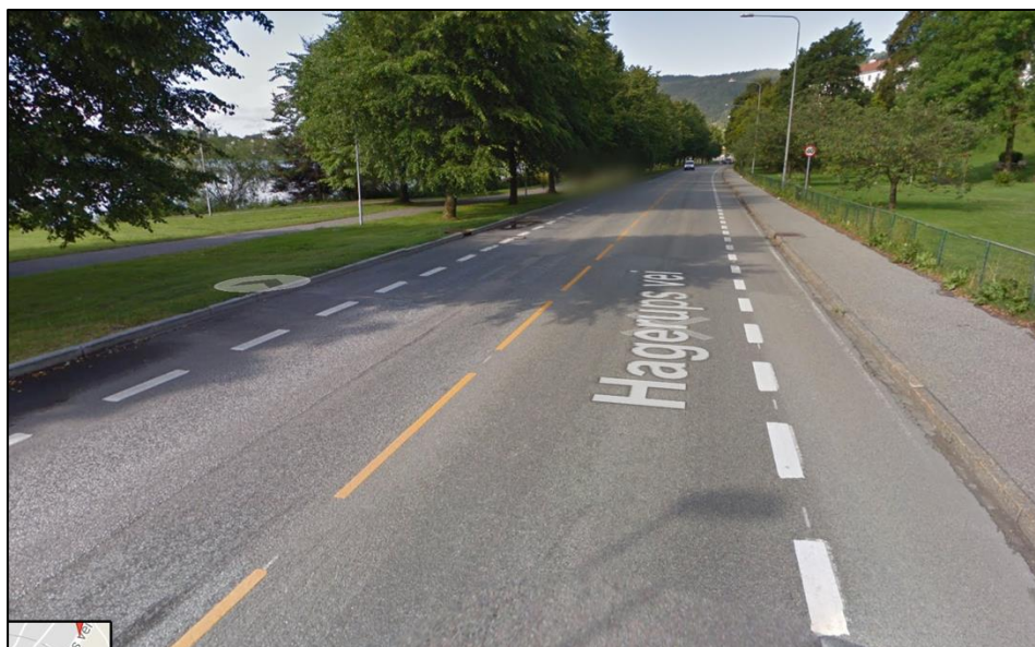
Figur 4: Hagerups vei, kilde: Google Street view
