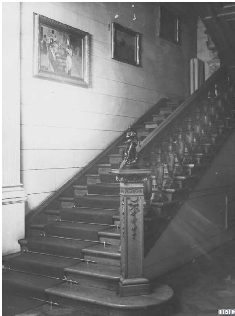
Fig. 6 Original side staircase.
